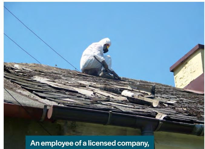
An employee of a licensed company, dressed in a white tight suit with an oxygen mask, sits on the roof and removes concrete-asbestos tiles
